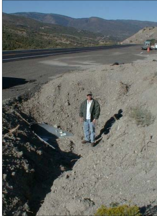
Soil eroded from the uplands accumulated at the mouth of this culvert.
